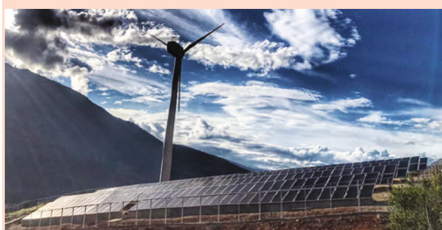
Capacity: 180kWp Location: Bhutan Power Corporation Rubessa-Bhutan
